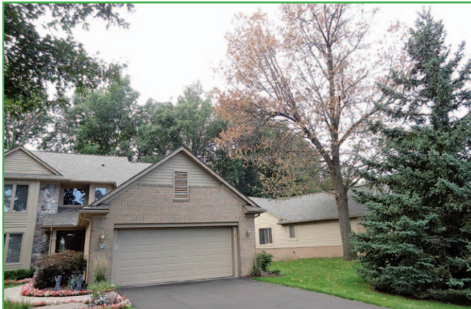
Photo 3: This tree contracted oak wilt when several small limbs were pruned from the tree because they supposedly threatened the roof of the nearby condo. In reality, a neighbor had convinced an elderly gentleman to prune this oak because he had wanted to defray his costs of removing two large oaks he had killed (oak wilt) behind his condo.
